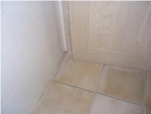
46. The toilet door binds on the floor, I think due to substrate movement.
