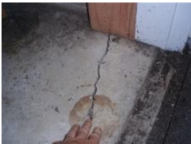
10. This shows the crack in the concrete floor. The floor has slumped noticeably.
