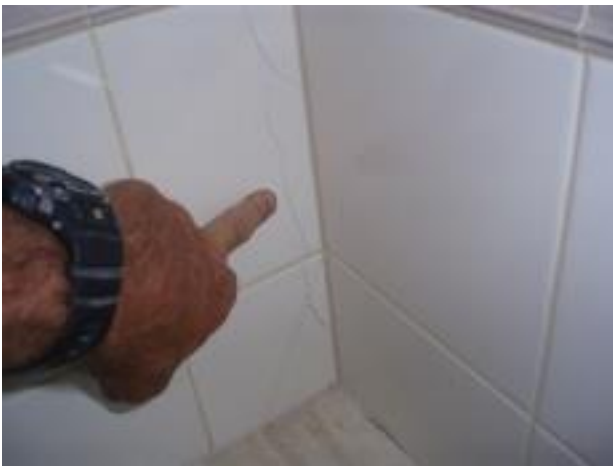
47. These cracked tiles, also in the bathroom, are probably also due to substrate movement.
