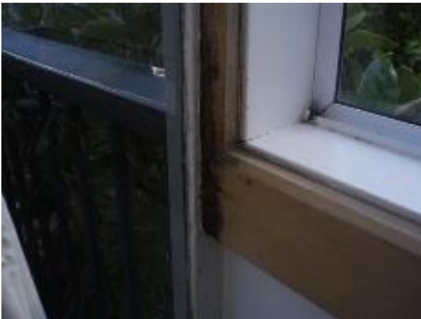
30. In the NE corner of the master bedroom the architrave of the window is discolored & moldy probably due to condensation around the steel window frame on the North wall.
