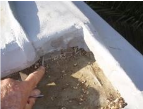
19. The entire roof has been covered with a paint on membrane but not a lot of attention was paid to detail & prep work. As an example I am pointing to a screw that was lying loose in the guttering & simply painted over.
