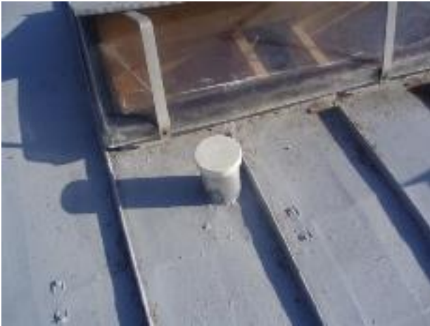
18. The roof has a lot of penetrations that appear to be superfluous.
