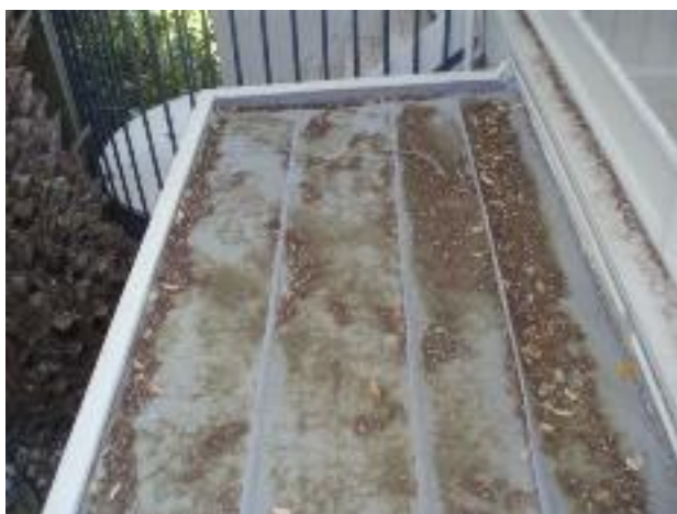
11. There is a lot of debris on the covered roof. It appears to leak & the gutter dropper (downpipe) is very small.
