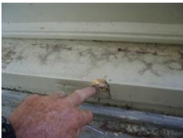
12. A decayed window sill on the Western wall of the lounge.
