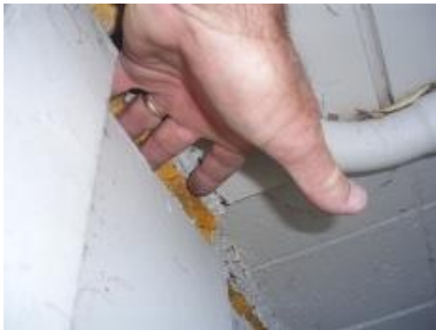
9. The concrete floor of the cupboard off the garage has settled causing this gap to open up.
