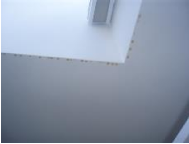
45. The discoloration around the edge of the skylight is caused by condensation / leaking.
