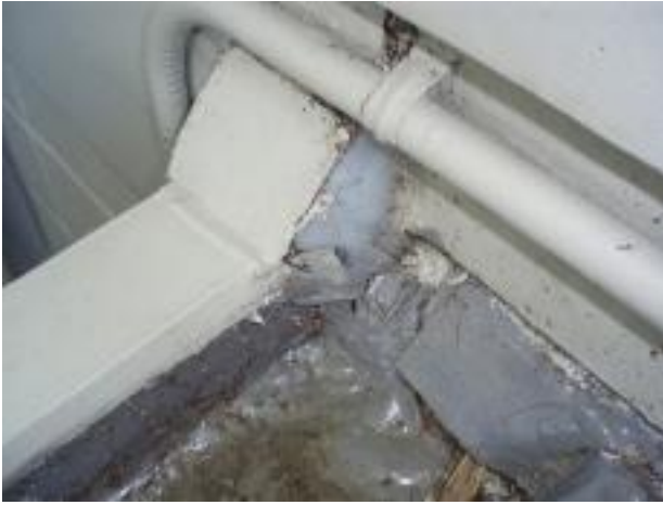
13. This junction of the cupboard roof to the cladding is not weathertight.
