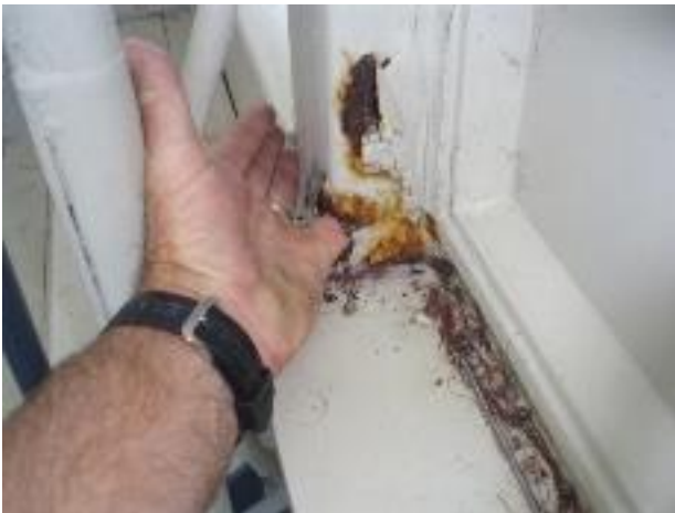
14. This shows severe corrosion of the SHS portal on the NW corner. You can see I have pushed my finger through the rust.
