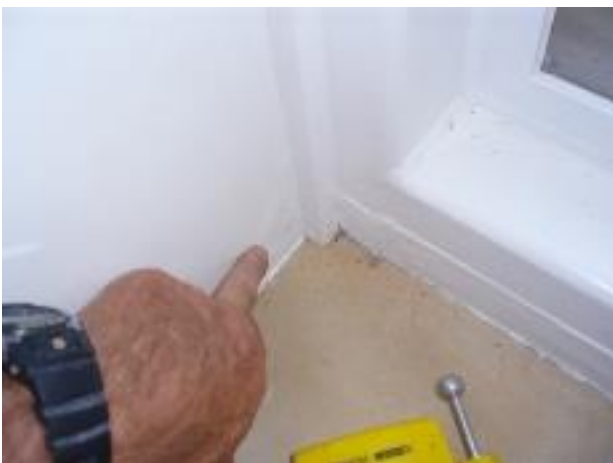
48. Water damage is visible on the gibboard wall in the entry lobby. The water ingress here may well stem from the steel portal highlighted in photo 2 & 3.
